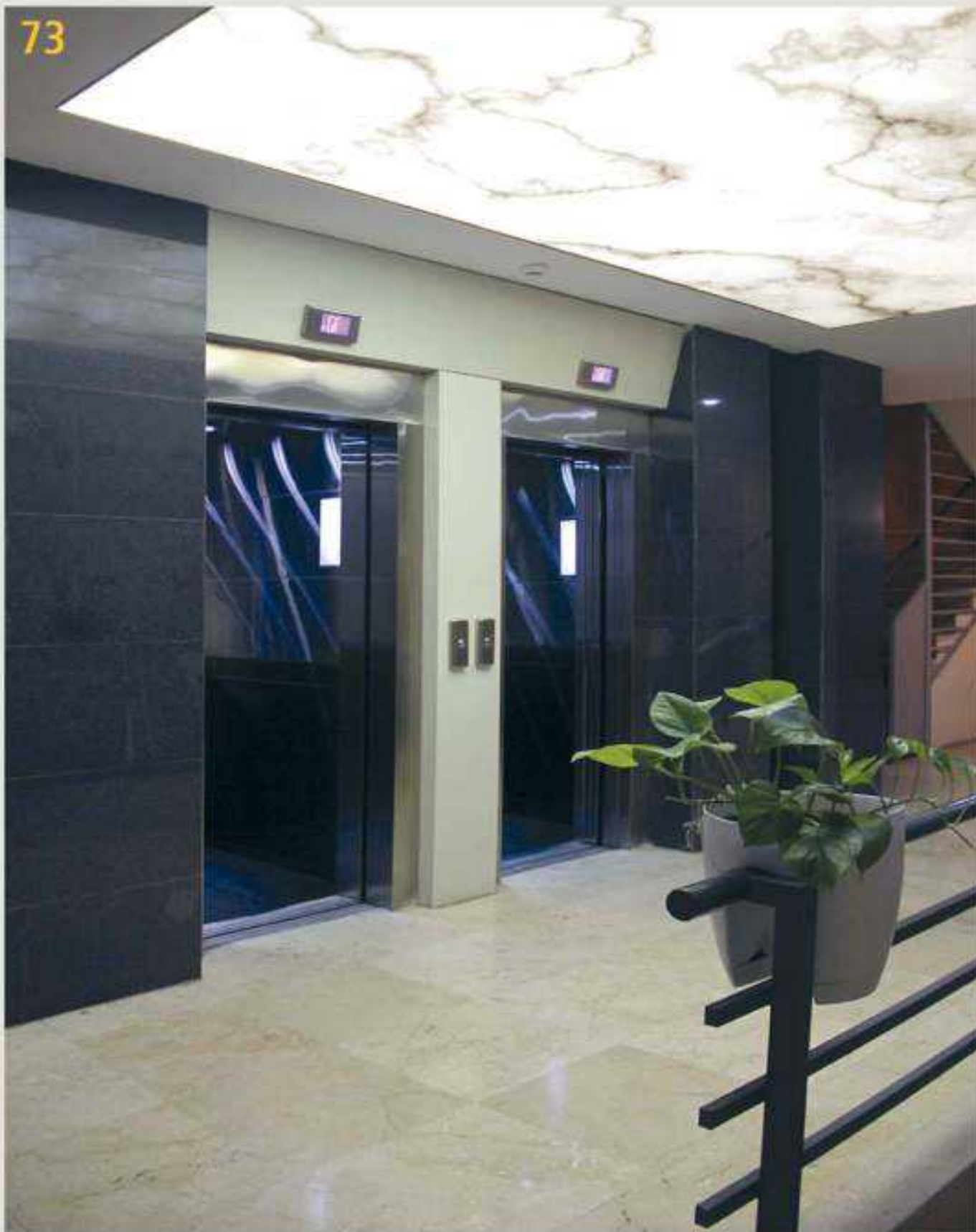
73 PROJECT NAME: UNIQUE OFFICIAL COMPLEX CLIENT: MOHAMMADREZA FERAYDOONI ELEVATOR TYPE: TRACTION - GEARLESS YEAR OF CONSTRUCTION: 2013/ 2014 NUMBER: 2 ELEVATORS
