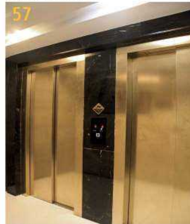
57-58 PROJECT NAME: DANA SARMAYEH OFFICIAL COMPLEX CLIENT: REZA SADEGHI ELEVATOR TYPE: TRACTION YEAR OF CONSTRUCTION: 2017 / 2018 NUMBER: 2 ELEVATORS
